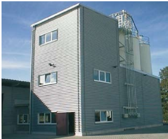
Fig. 4.1: External view of the Hydroment plant
