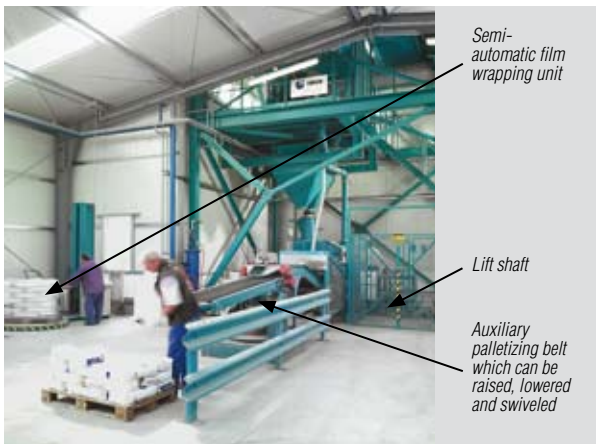
Fig. 3.2: Manual palletizing with auxiliary belt
