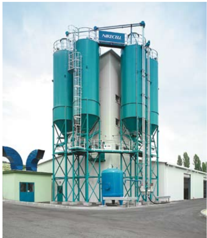
Fig. 2.1: External view of the Nikecell plant in Hungary
