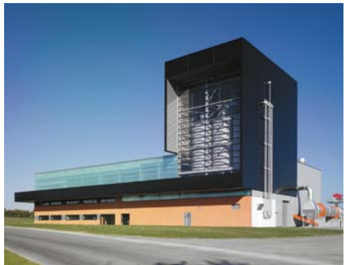
Fig. 4.4: External view of the Egid plant
