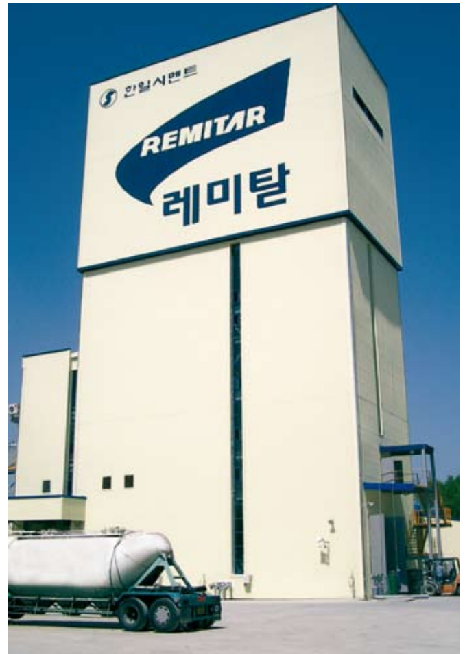
Fig. 5.2: External view of the Hanil Cement plant
