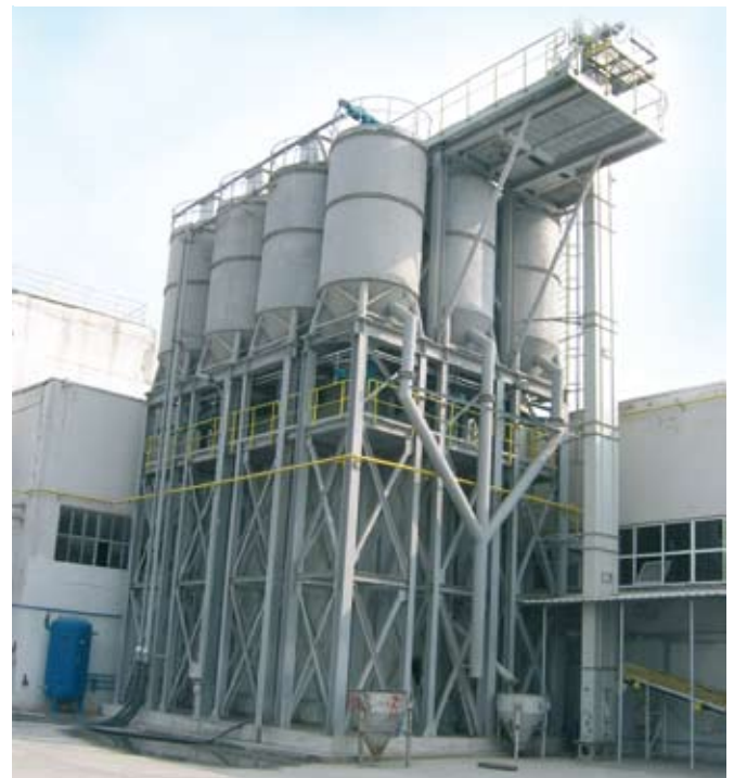
Fig. 3.4: Top view of the Celco plant, Romania
